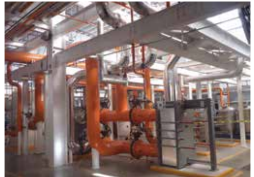
Plate and frame heat exchanger for weld water
