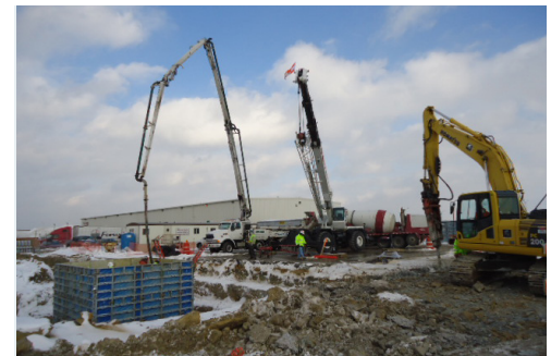
Construction of Mechanical Vault A
