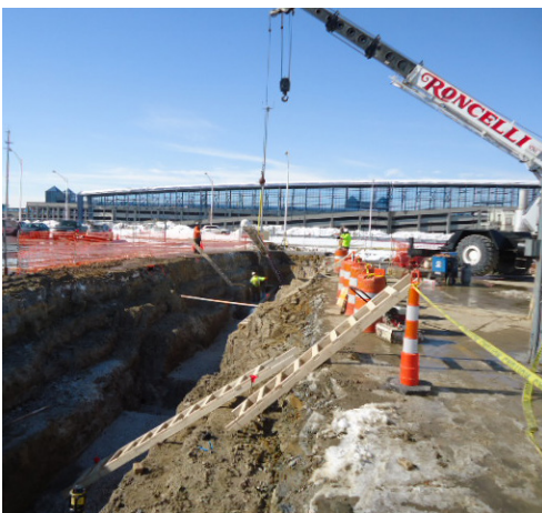
Installation of containment piping
